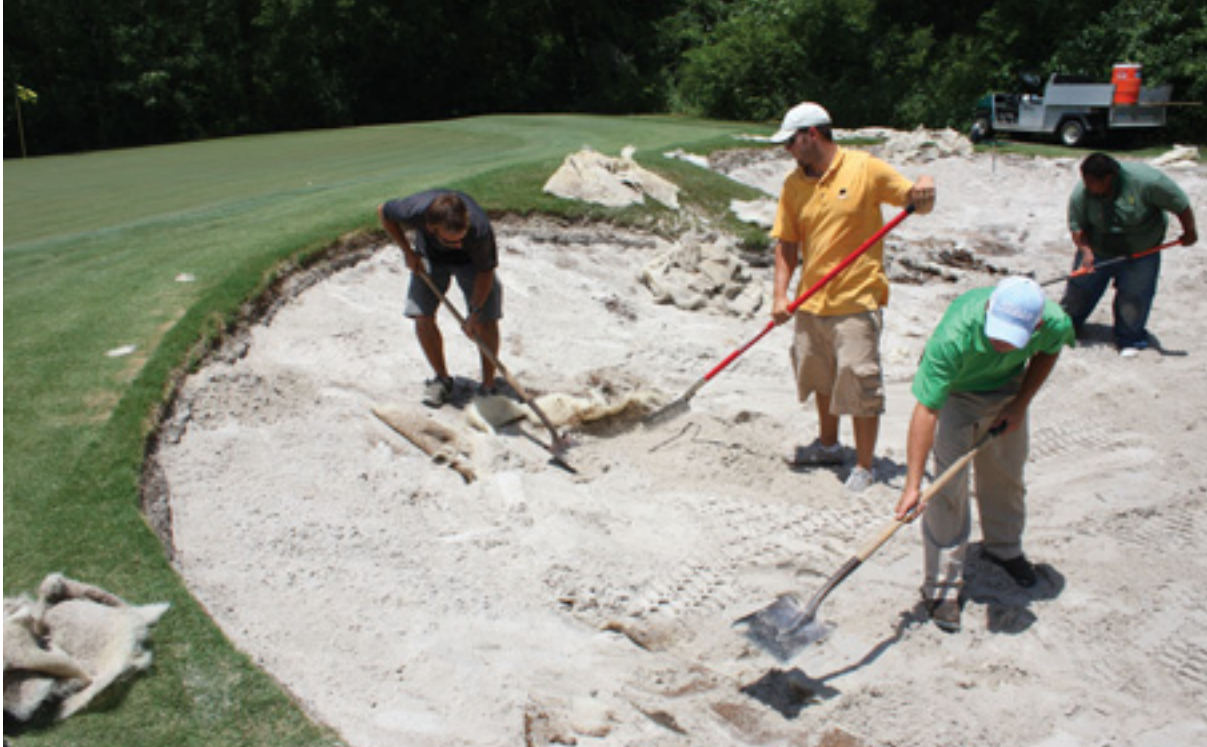
Bunker liners are not a cure-all. Unless a great deal of labor is expended to keep plenty of sand on the bunker face, the liner can become exposed and snagged by golfers. To prevent maintenance equipment from damaging the liner, labor-intensive hand-raking of bunkers is recommended when liners are used.
