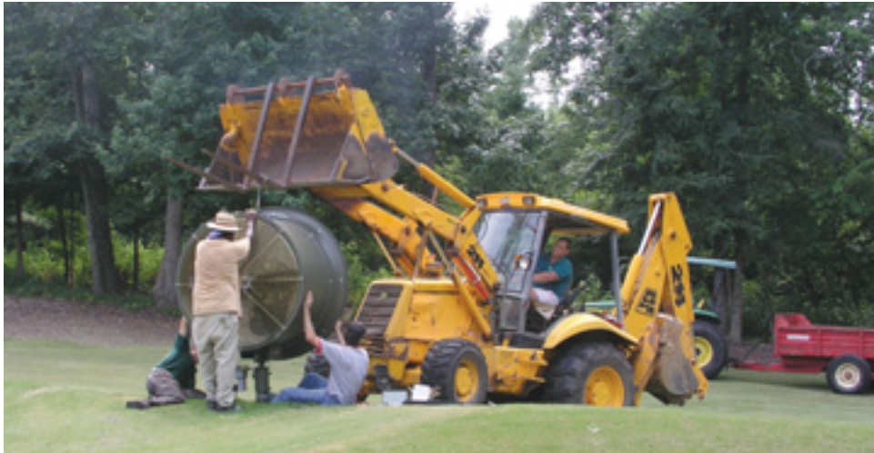
A backhoe or front-end loader easily lifts the fan for assembly to the fan pole. A fork attachment on the loader is a plus to help lift and maneuver the fan. Remember, some type of device also will be needed to transport the fans on and off the golf course for off-season storage.
