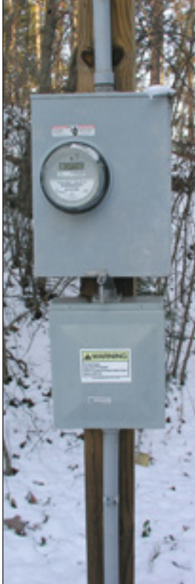
Above left: As the primary power for the fan, the power company's electric meter and breaker master switch are located on a pole close to the putting green. Wire from the power supply takes either single-phase or three-phase power to the fan. Top right: Timers are sometimes mounted in a box, either on the fan pole or near the fan to modulate fan operation times. Above right: Weatherproof covers are used to protect the fan motor and belts during the off-season when indoor storage facilities are not available.
