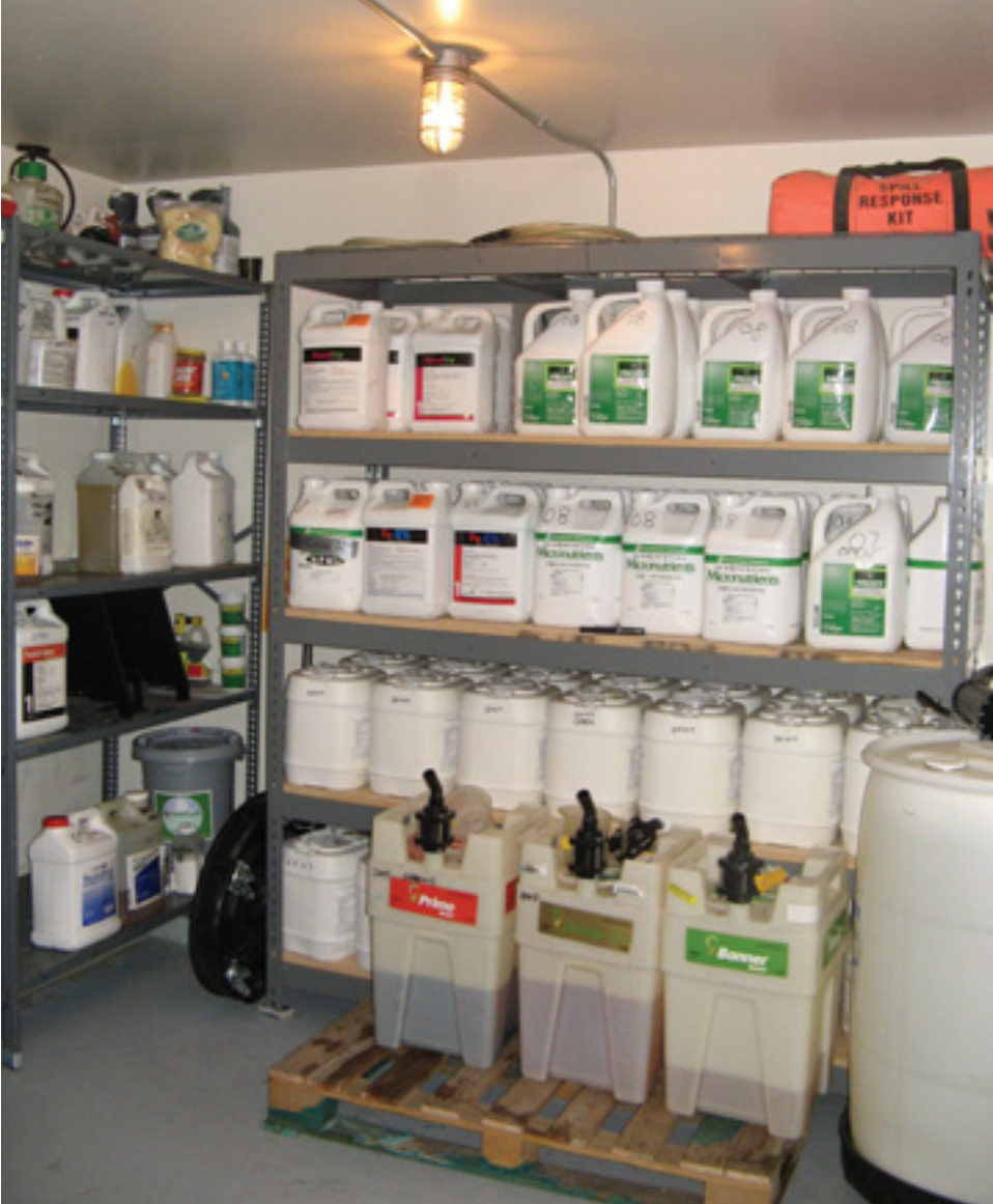
In this maintenance facility, the spill kit is located behind large containers and is too high to be removed quickly. Keep spill kits near the entrance and easily accessible in case an accident does occur.
