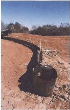
30 ml plastic can be purchased that makes the installation easier due to the stiffness of the material.
