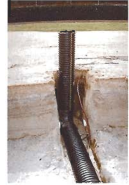
Exit the wire near the "clean-out" or near a sprinkler so the end of the wire can be found easily.
