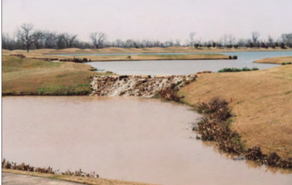
Water will be diverted into the pond in the foreground. Multiple ponds can be interconnected for increased storage. Water transfer can be creative and add aesthetic features to the course.
