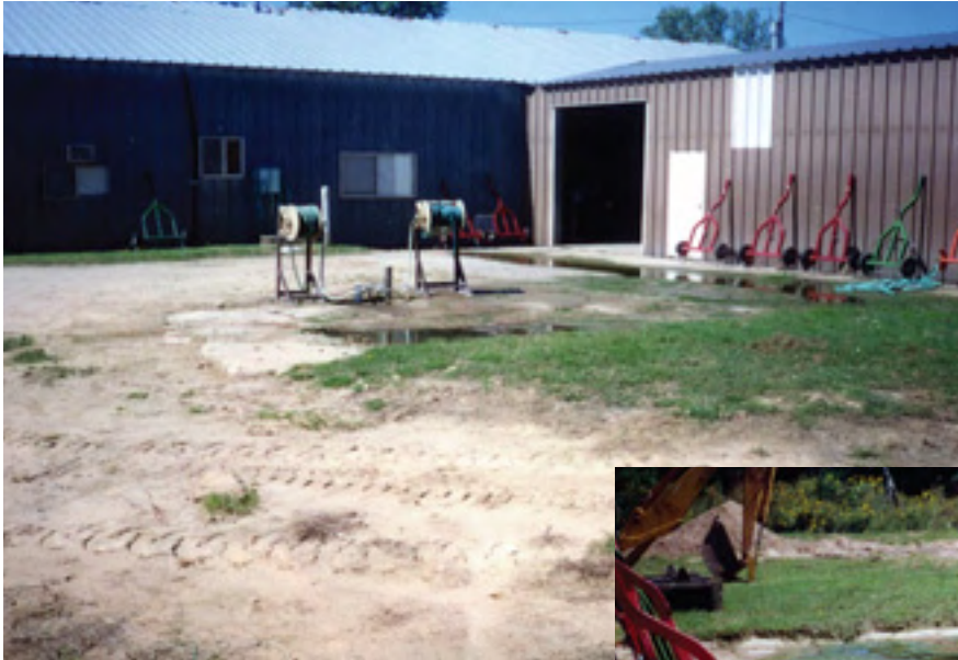
Failing drains and stagnant water plagued Prairie Dunes Country Club's wash pad before the upgrade.
