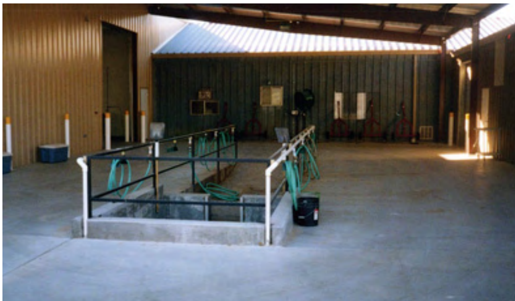
The redesigned and greatly improved wash pad at Prairie Dunes Country Club provides adequate collection and filtering of wash water.
